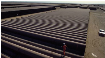
Pipe yard in Yanbu (history, 1982)
